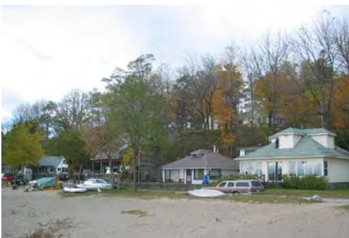
The cottages built on beach front are subject to flooding and erosion.
