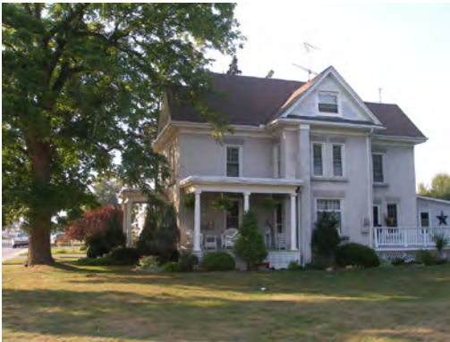
A collection of large traditional homes serve as a gateway to the commercial core approaching from the north on Bay Street.
