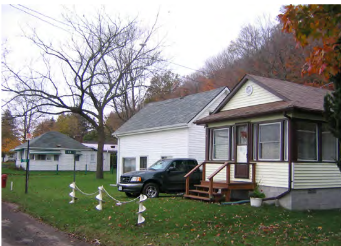
Typical scale of older cottages in Turkey Point.
