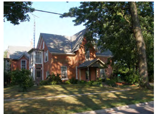
Older Gothic farmhouse on Townline Street.
