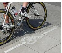
(Left) Bicycle Signal Loop Detector Stencil Pavement Marking, (Right) Example Pavement Marking for Bicycle Actuation Location Source – T.A.C. Bikeway Traffic Control Guidelines, 2012
