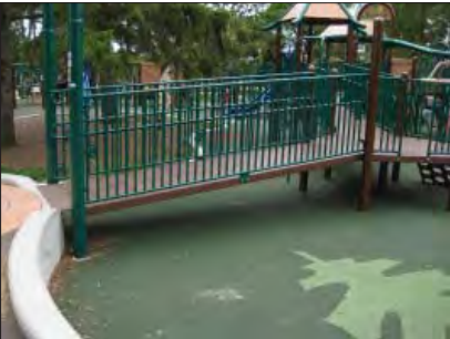
Ramp connected to elevated play components.
