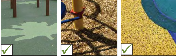
Examples of inclusive play space ground surfaces. From left to right: poured-in-place rubber, engineered wood fibre and shredded rubber.
