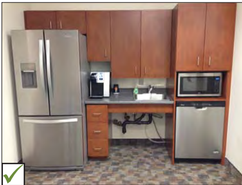
Accessible counter space and sink with knee clearance.
