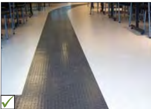
Example of tactile floor surface to guide users with vision loss (Best Practice).
