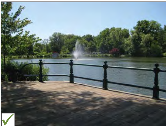
Example of protective barrier where there is a large elevation change or trail is adjacent to water feature.
