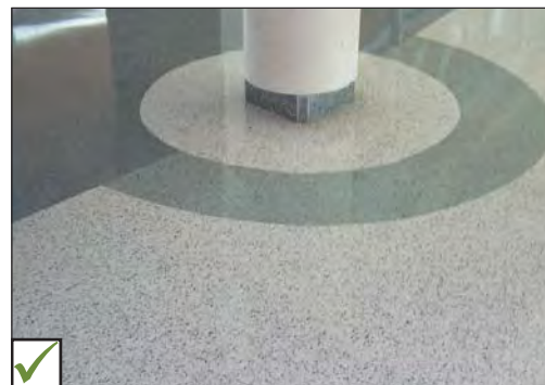
Where a structural column / support may be within an accessible route, a colour contrasted floor surface at base helps identify its location to prevent a potential bumping hazard.
