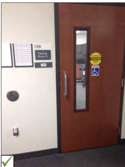
Example of power door operator control mounted at suitable distance from floor swing.
