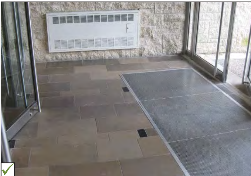
Example of a recessed floor mat system which is preferred.
