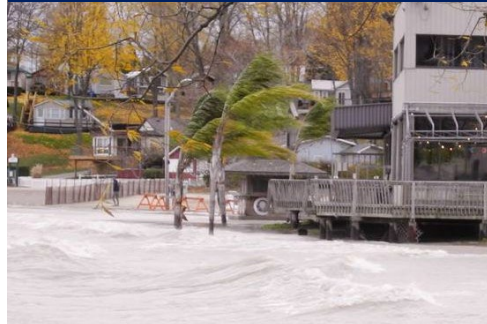
Flooding and shoreline road closures 100km/hr wind gusts November 2018
