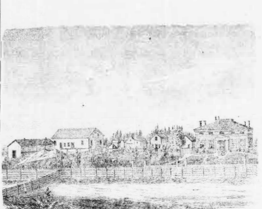
Residence of JAMES L. GREEN Esq. Waterford.
