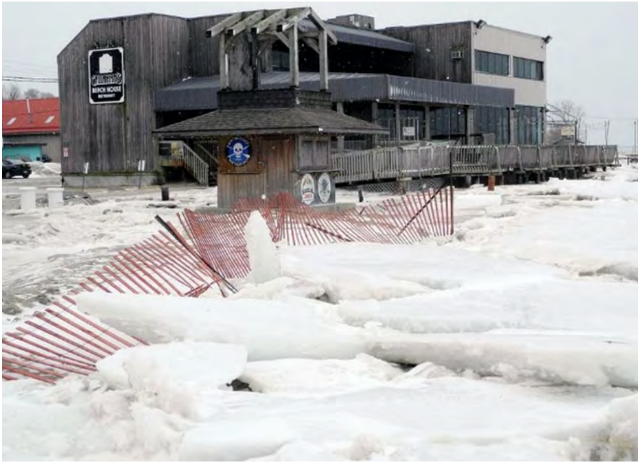
Figure 6.9: Ice pile-up along Walker St. in Port Dover, at The Beach House looking East (Sonnenberg, 2019)
