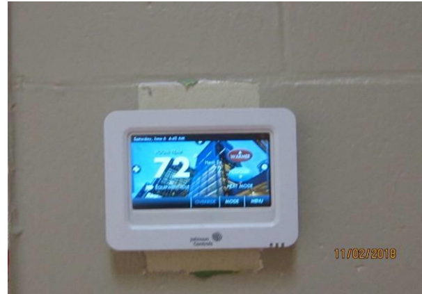
View showing the condition of the new thermostat in the building.
