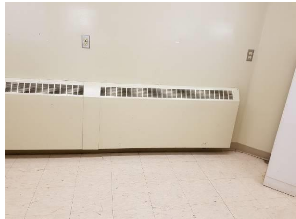
View showing typical condition of the baseboard heaters in the building.
