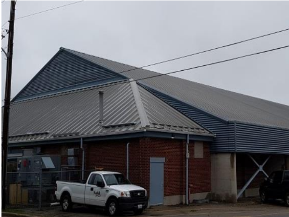
View showing the metal cladding at the building perimeter and gables.
