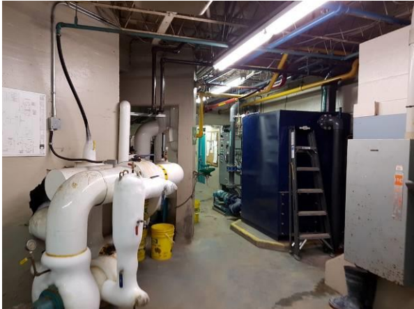
View showing overall condition of the refrigerator room.
