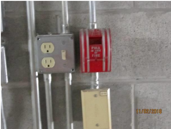
View showing the condition of the pull stations.
