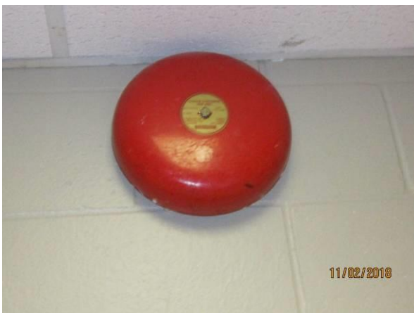
View showing the condition of the fire bell.
