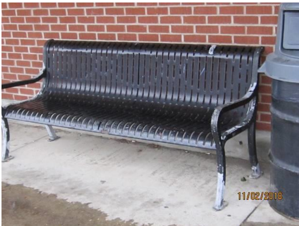
View showing the condition of the metal bench near the main entrance.
