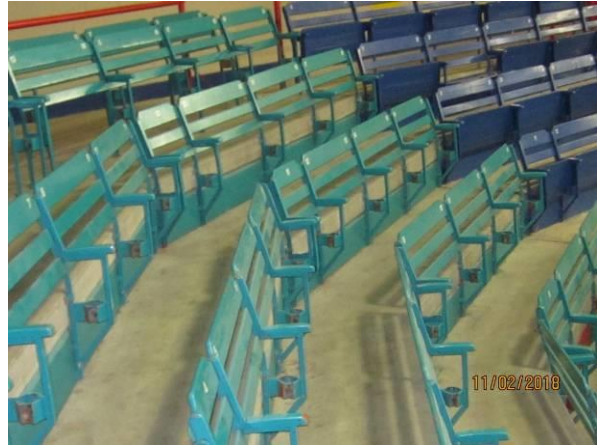
View showing damaged/missing wood seats in the Arena.
