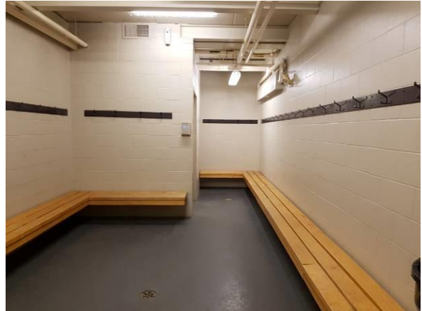
View showing the condition of the wood seats in the change rooms.
