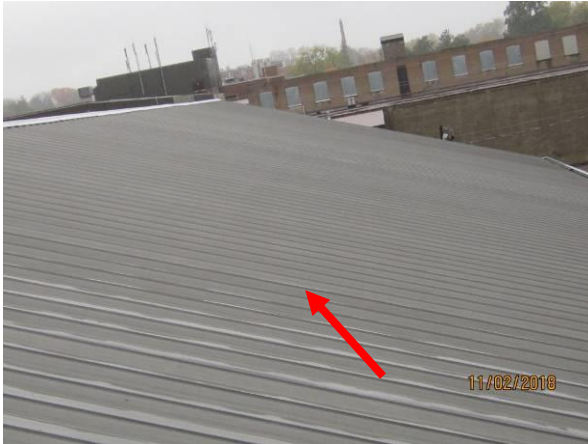
View showing the overall condition of the sloped metal roof.
