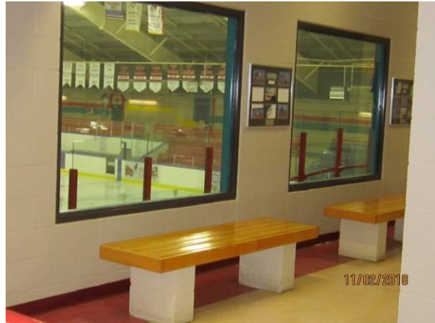
View showing typical condition of the interior window assembly.
