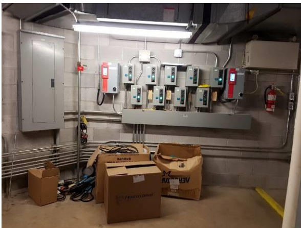
View showing the condition of the electrical panels in the penthouse.
