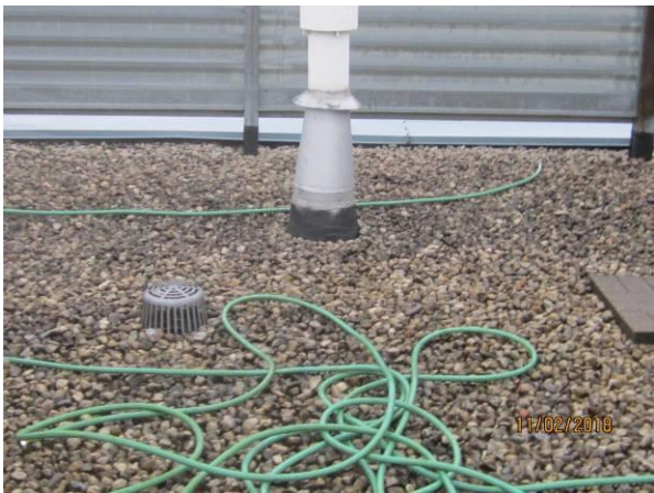
View showing the overall condition of the flat roof.
