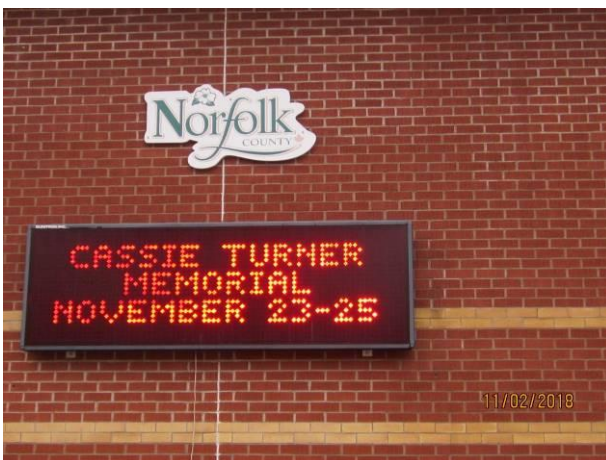
View showing the condition of the wall mounted building's main sign.
