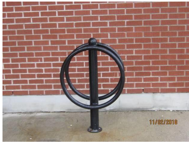
View showing the condition of the bicycle rack located near the main entrance.
