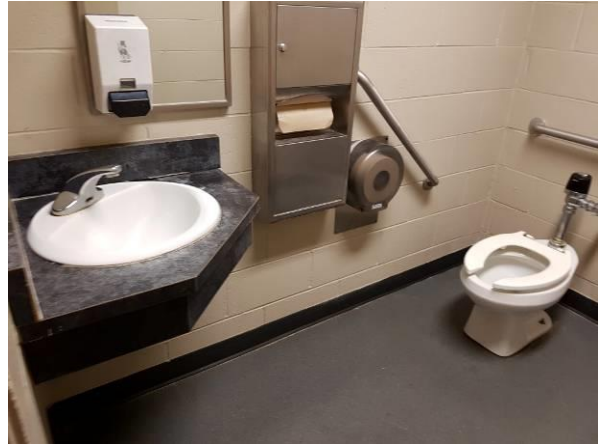
View showing the condition of the accessible washroom.
