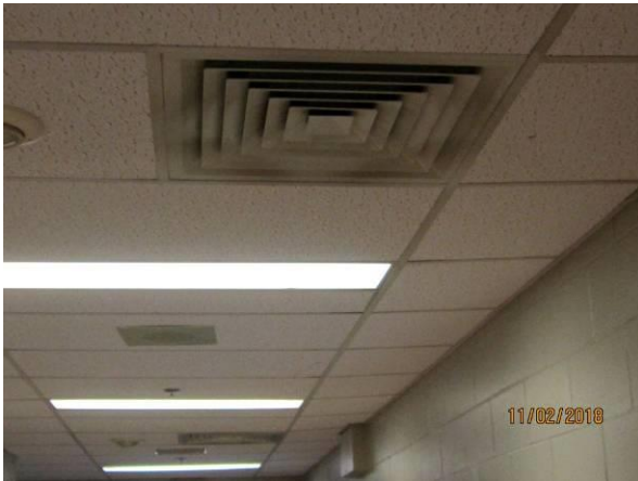
View showing the condition of the interior lighting.
