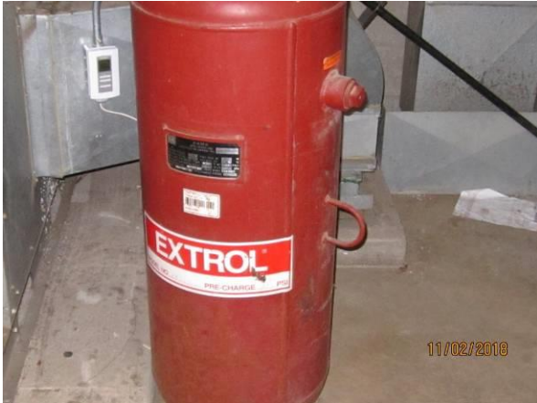
View showing the condition of the pressure tank in the penthouse.
