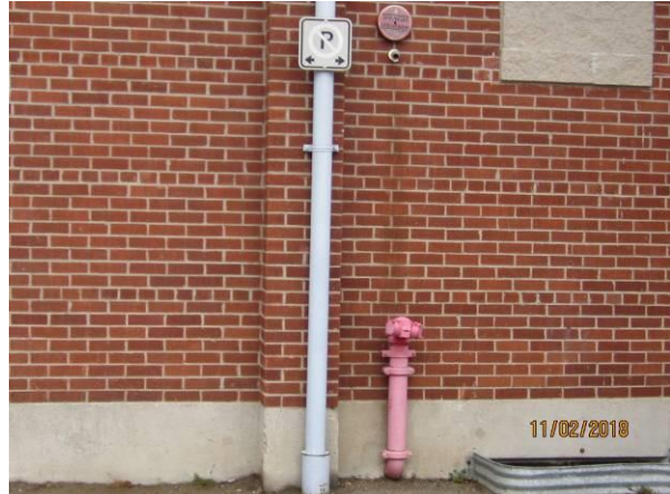
View showing the Siamese connection at the south elevation.
