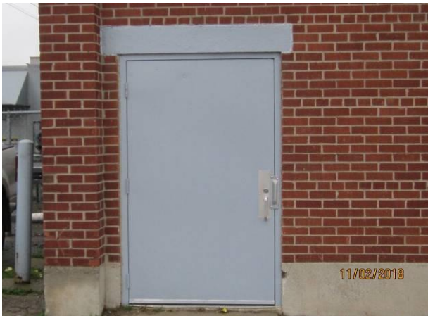
View showing overall condition of the metal single service door.
