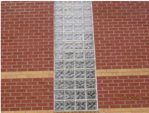
View showing the condition of the brick veneer.
