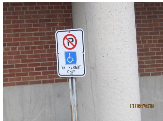
View showing the condition of the site signs in the parking lot area.
