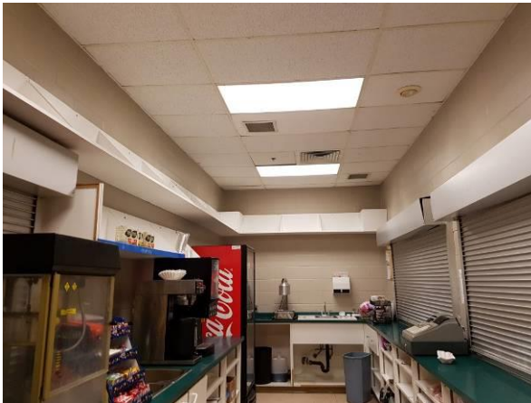
View showing overall condition of the drop down ceiling.
