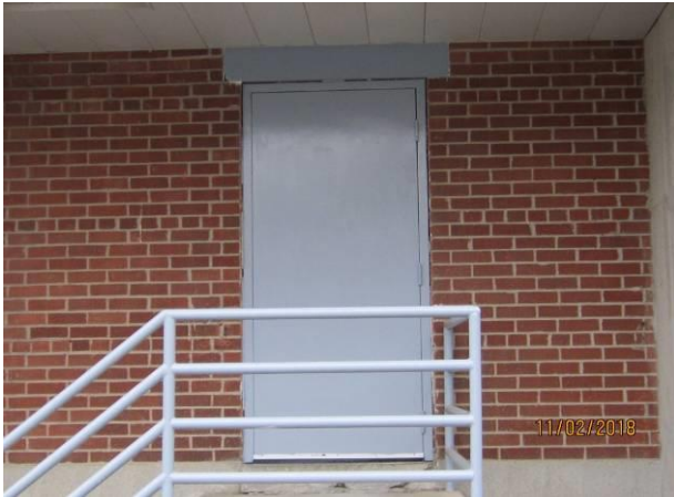
View showing the condition of the exterior single leaf door.
