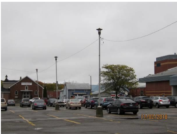
View showing the condition of pole-mounted exterior lighting in the parking lot.
