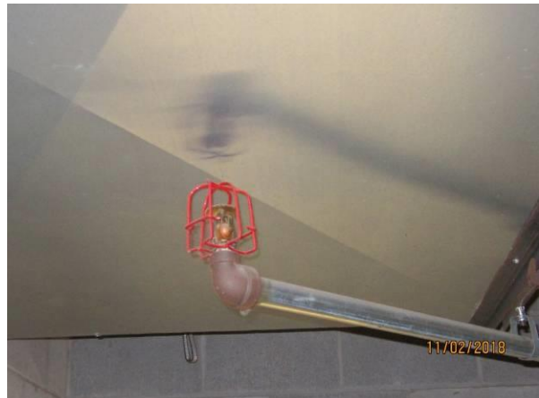
View showing the condition of the sprinkler heads.
