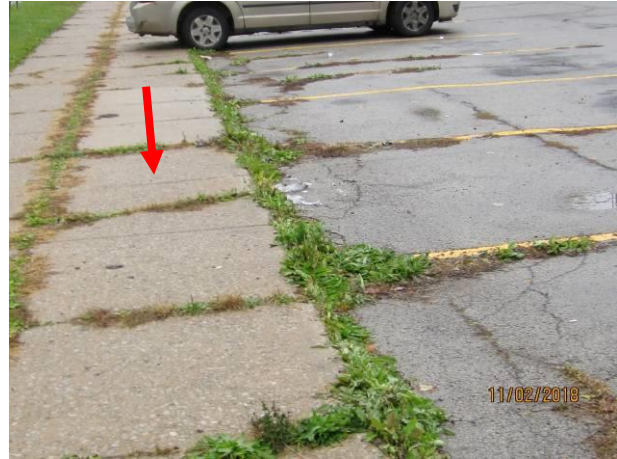
View showing broken, uneven with growing vegetation in the walkway at the west side of the property.
