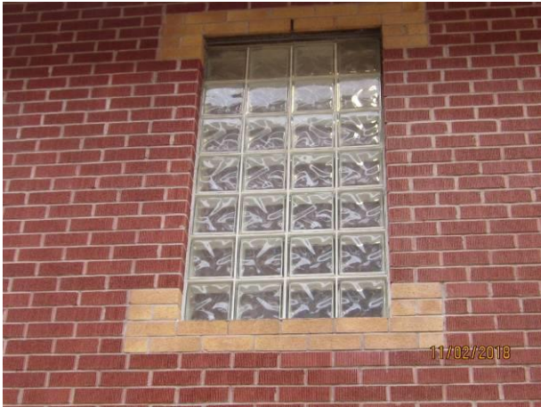
View showing typical condition of the exterior window assembly.
